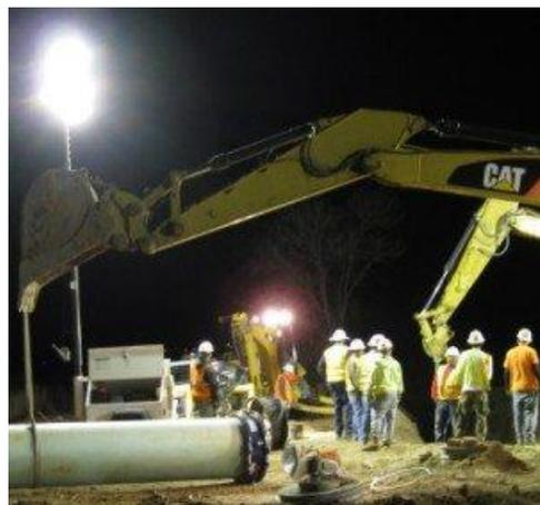
Make sure everything is done with a focus on safety. This includes wearing reflective clothing in accordance with the law, and using a trench box or shoring to ensure that the trench doesn't collapse while workers are inside. There are many who never use a trench box because it gets in the way of some repairs. At night, the use of trench boxes and shoring is even more critical. Make trench boxes a normal part of every excavation, and never put speed ahead of safety.
